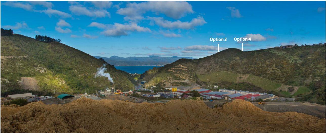
Approximate locations of the maximum extent of the quarry area cuts under options 3-4
