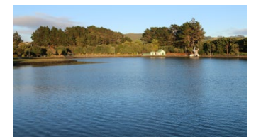
Aotea Stormwater Pond Porirua
