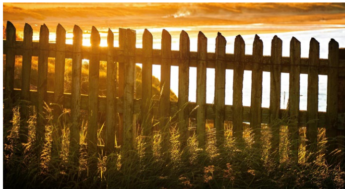
Picket fence with pickets or palings spaced a minimum of 50mm apart and with a 150 mm clearance off the ground
