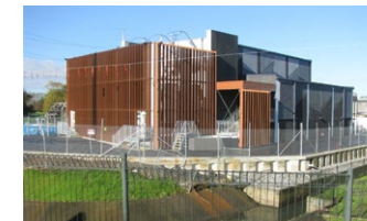
Wairau Road substation Auckland Image courtesy of Transpower
