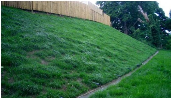
Contour drain. Source: ResearchGate
