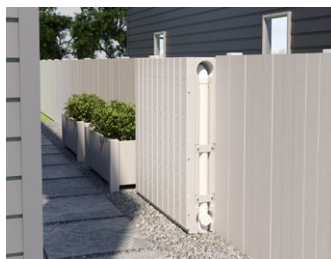
A 1000L rainwater tank fixed to a fence Image courtesy of Watersmart
