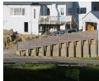
Retaining wall with wall made of timber
