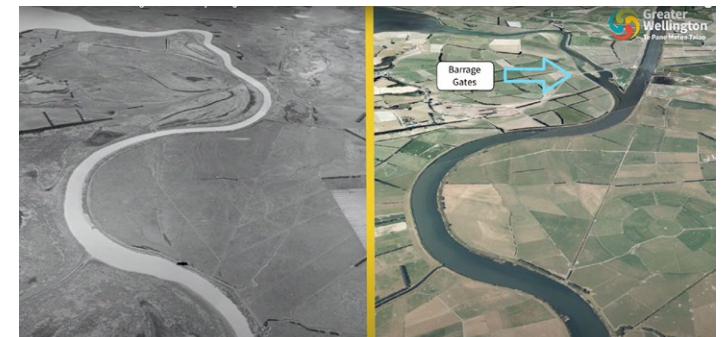
Ruamahanga River diversion channel (to the right of the barrage gates) as part of the LWVDS, diverting water from its direct course into Lake Wairarapa to prevent flooding
