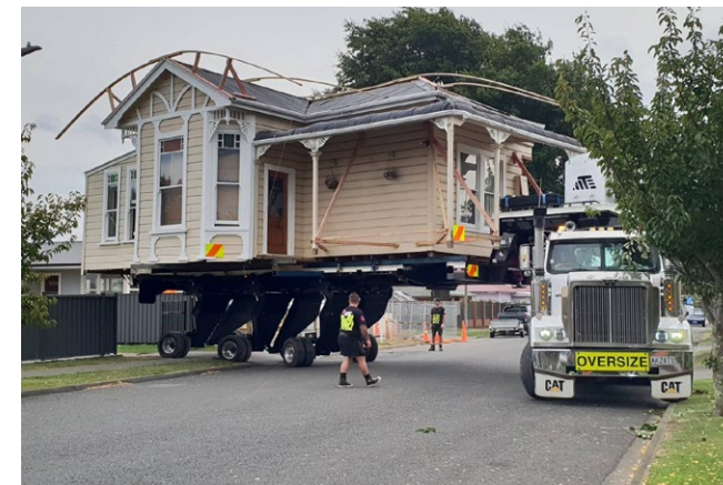
Relocating a house
