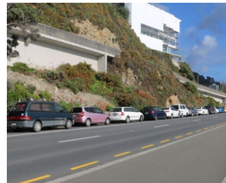
Carlton Gore Road and Retaining Wall
