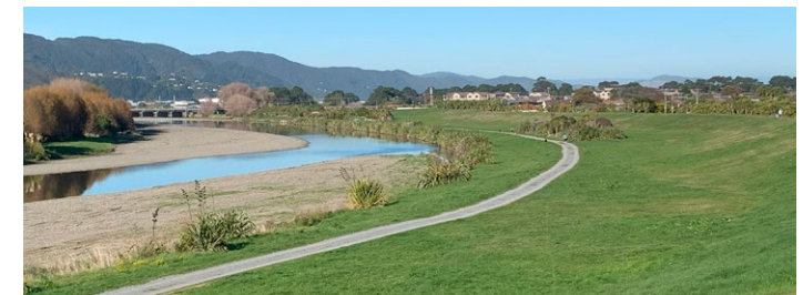
Stop banks along Te Awa Kairangi/Hutt River
