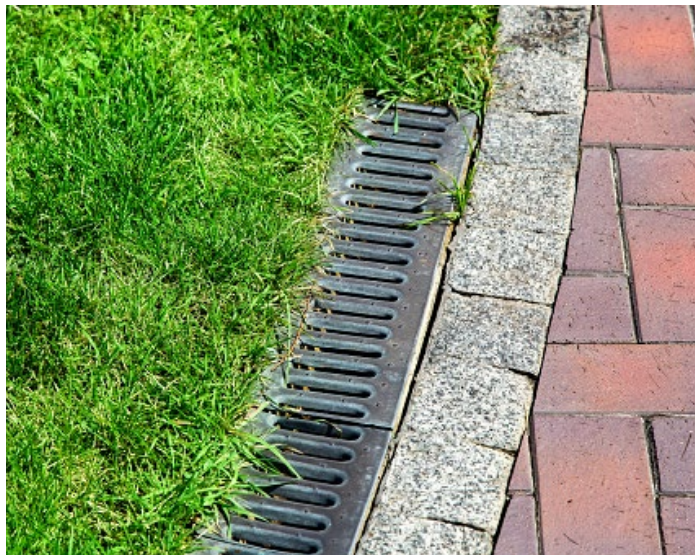
Backyard drainage system
