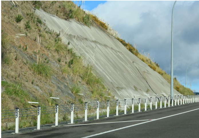
Underground slope drainage on Transmission Gully
