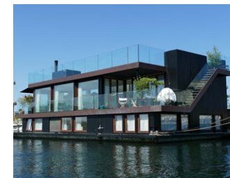
A modern floating house
