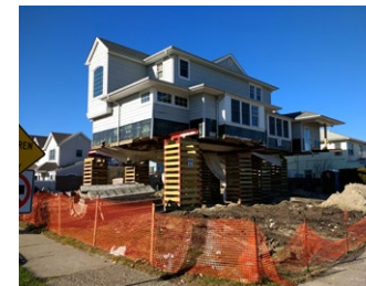
House being retrospectively raised
