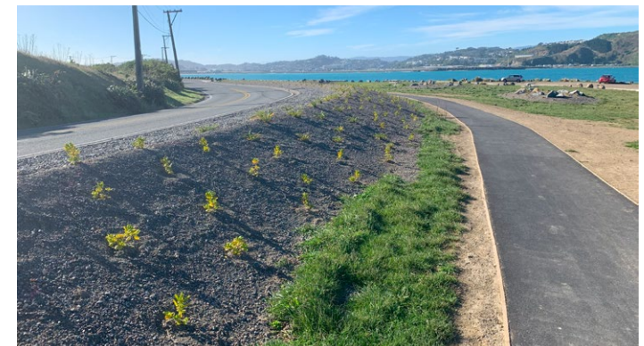
Gravel bund on Wellington's South Coast
