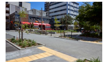
Swan Lane rain garden Image courtesy of JFC Ltd
