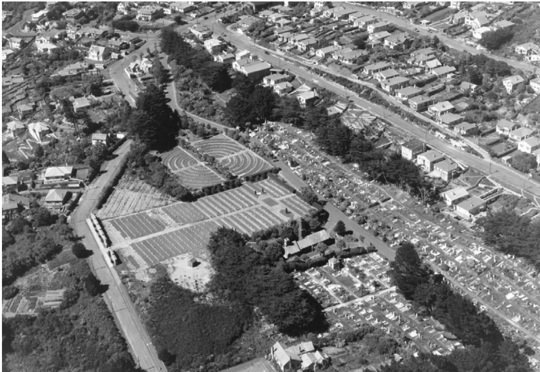
An aerial image of the area near the cemetery entrance, taken from the north, 1947. The future site of the main chapel and Services Cemetery extension is in the foreground. (WA-11396-F, ATL)
