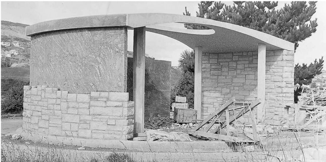
The Peter Fraser memorial nearing completion, 1956. (EP/1956/0644-F)
