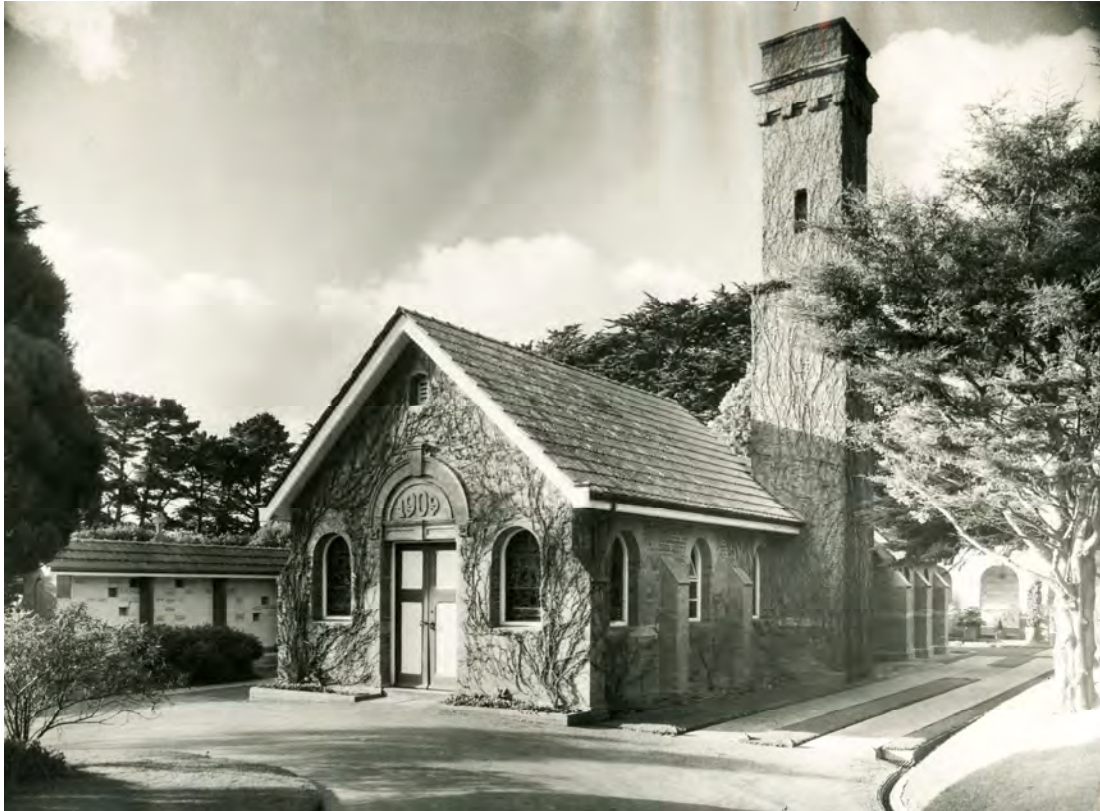
The chapel and crematorium, with the 1949 columbarium behind, left, and the original 1935 columbarium, right (rear). (Date unknown, likely early 1950s, 50003-410, WCCA)
