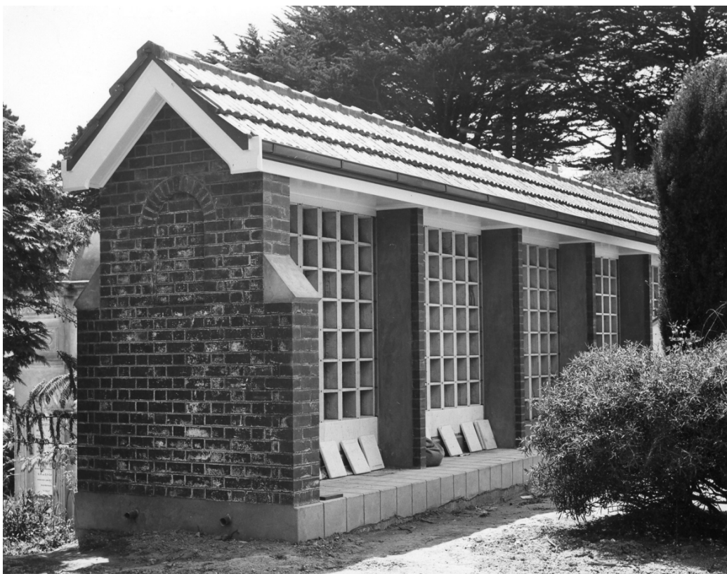
The stand-alone columbarium nearing completion alongside the chapel/crematorium, 1950. (00009_7;2;1 Part 1, WCA)
