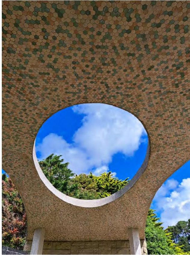
The ceiling of the Peter Fraser Memorial.
