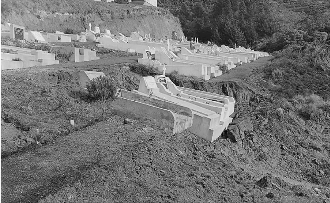
Graves slowly sliding down a slumping hillside, north end of the cemetery, 1956. (EP/1956/1521-F)
