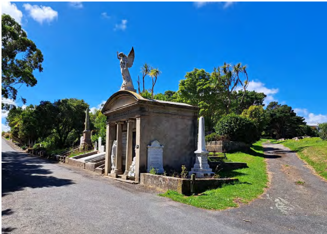
The Underwood vault, just north of the Shelter, an example of one of the cemetery's 24 vaults.
