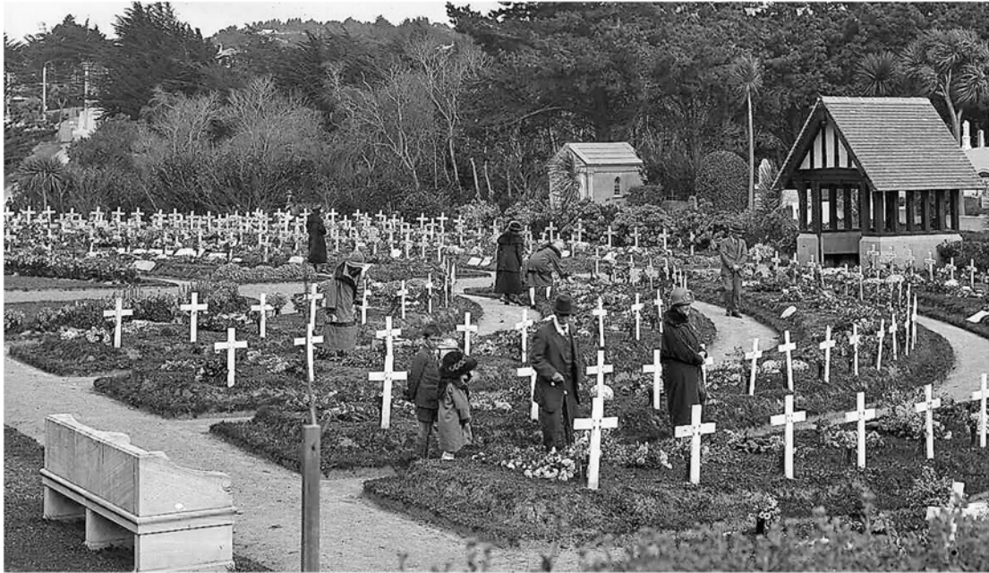
The Services Cemetery taking shape, with marble seats and lychgate, c.1921. Memorial objects such as these were used to help beautify the cemetery. (50010-57, WCCA)
