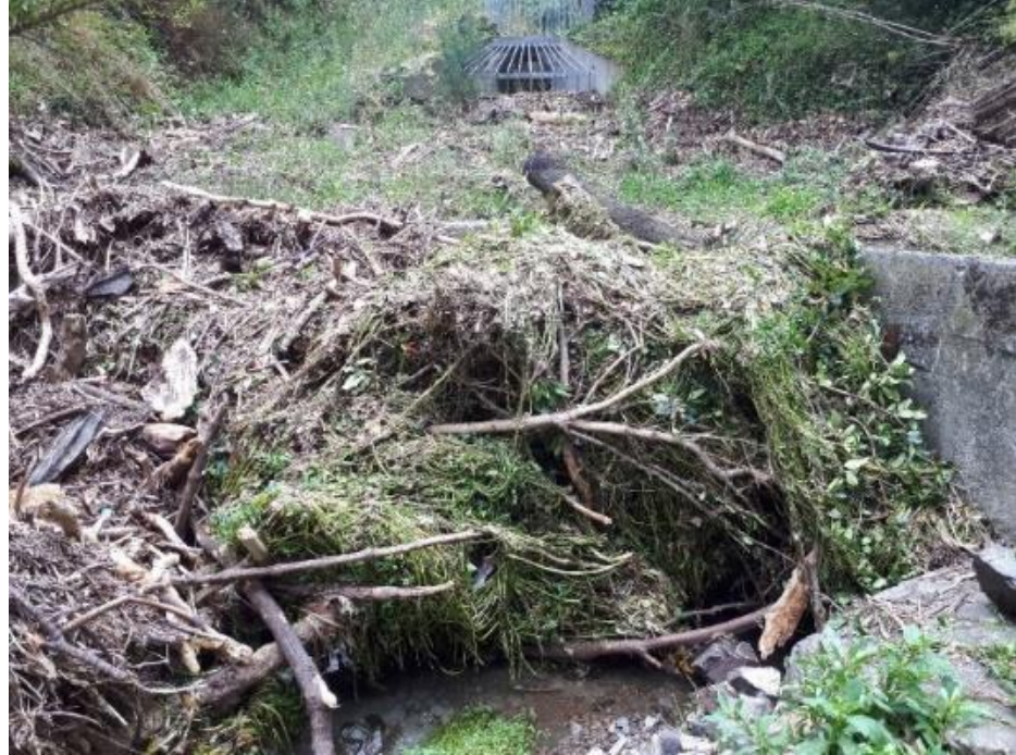
Stormwater grills blocked after severe rainfall event, leading to an increase in downstream flooding and blocking of fish passage to the sea.
