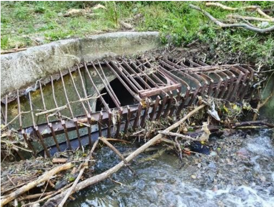
Stormwater grills blocked after severe rainfall event, leading to an increase in downstream flooding and blocking of fish passage to the sea.
