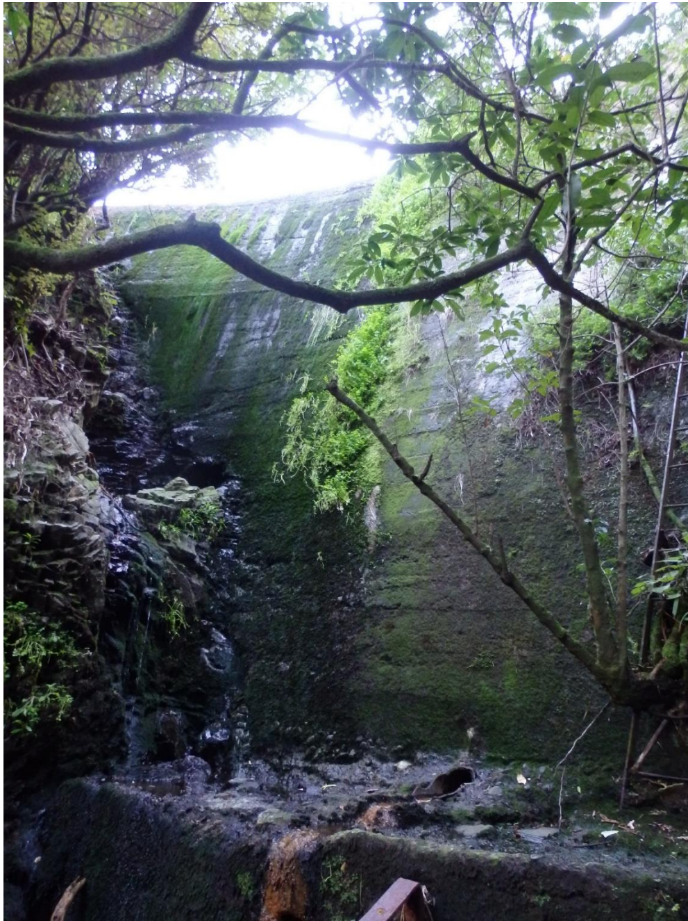
6 Tyers Stream Dam
