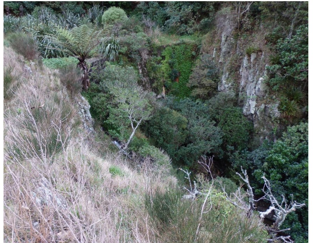
7 Tyers Stream Dam
