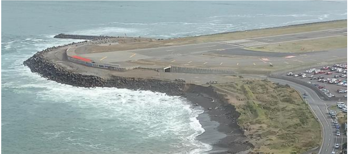
Figure 2 – Image showing general layout of existing site components, being the Southern Seawall, eroding Eastern Embankment and modified dunes.
