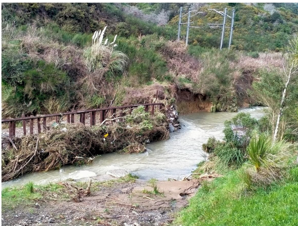
Debris Arrestor, Middleton Road, 18 July 2021 (Porirua Stream)
