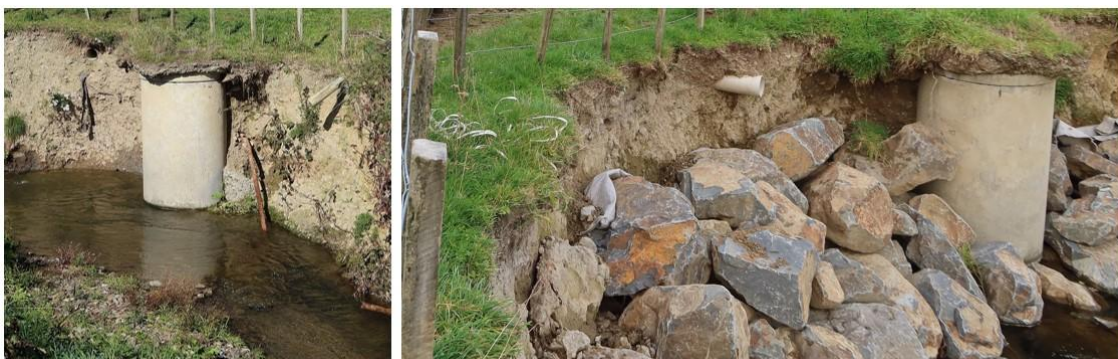
Erosion around sewer shaft in Glenside Reserve brought to attention Wellington Water in 2023 (left) and the attempt to mitigate exposure (right).
