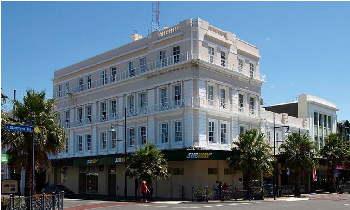
Seized building: Gisborne's Masonic Hotel (now closed) prior to its decline. 46 Gladstone Rd
