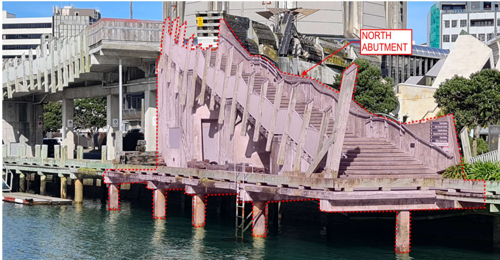
Figure 3: Photograph shown the North Abutment
