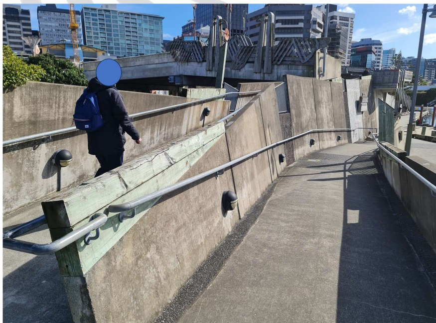
Figure 4: Photo of the South Abutment ramp
