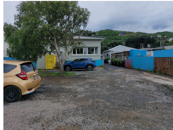
4. View NNW - Rear of library, Silver Birch left centre.
