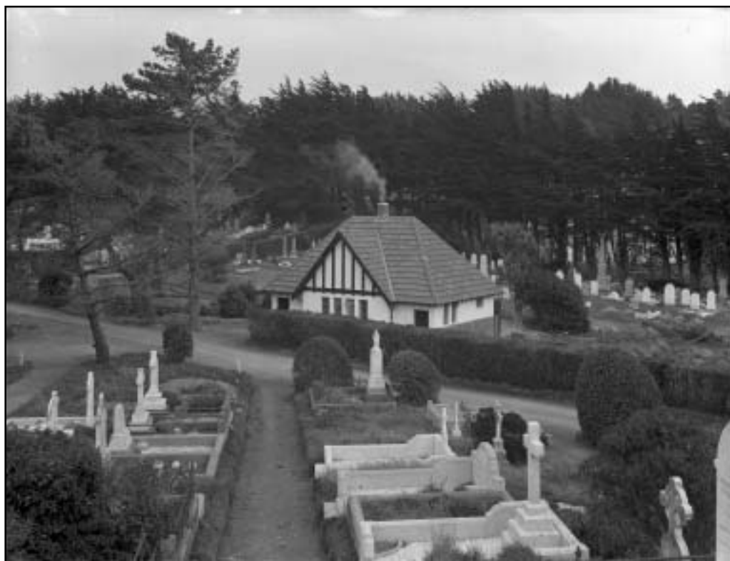
Figure 15: The Mess and Toolshed in 1927 soon after its completion (and before its additions) reveals the quality of the City Engineer's building designs. The growing macrocarpa and pine trees were by then becoming a maintenance issue. (ATL G247521 1/1)
