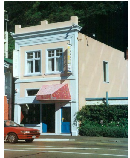
Ground level activities that support the public use of the area
