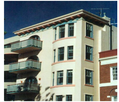
Balconies on front elevations provide private open space and enhance the “public face” of buildings
