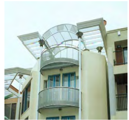
Distinctive building top adding interest to the silhouette line
