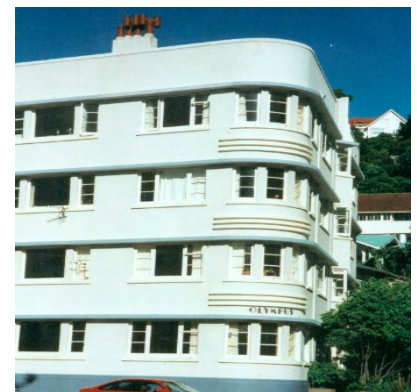
Floor to floor height and window openings useful indicators of scale
