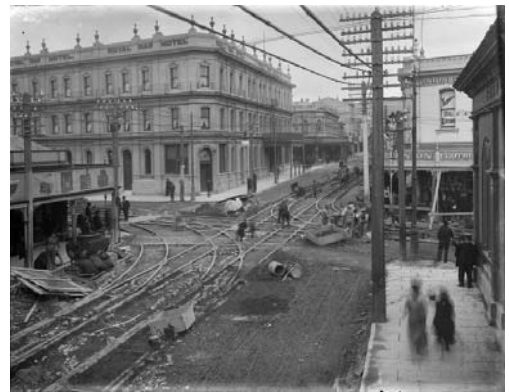
Laying of tracks for the electric tramway, 1903, at the intersection of Manners and Cuba Streets. The still newly constructed Royal Oak is in the immediate background, with the Union Clothing Co. on the other side of the road. (G002130-1/1, ATL)
