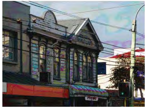
Upper level windows and parapets
