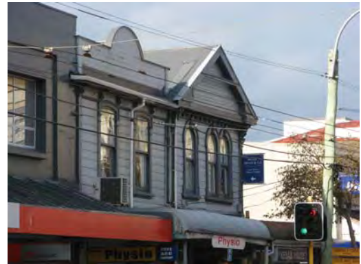
Upper level windows and parapets
