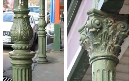
Detail of cast iron veranda posts
