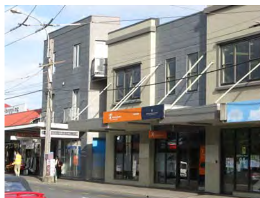
Some recent buildings contribute positively to the streetscape
