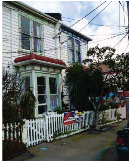
Neighbouring buildings, aligned with each other give a strong street edge definition
