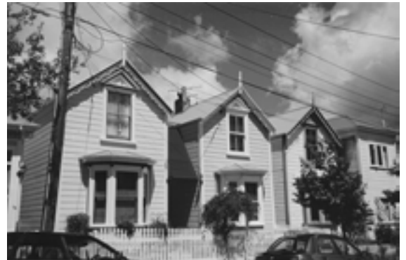
The Cottage is another recurring building type
