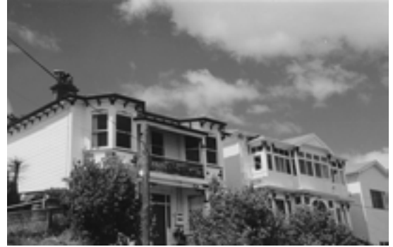
Painted weatherboards and corrugated iron are the predominant materials.
