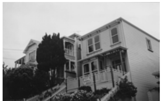
Group of two storey villas in contrast to the predominant setting of single storey dwellings
