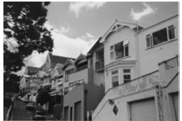
McFarlane Street (eastern side) – a notable collection of original dwellings
