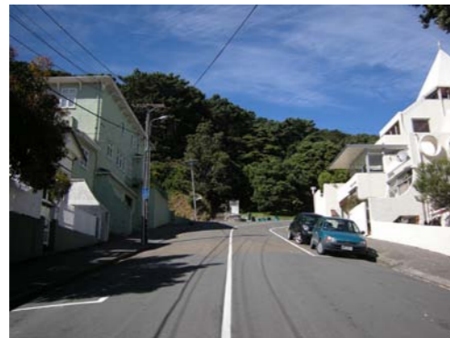
Figure 10. Existing Majoribanks Street.
