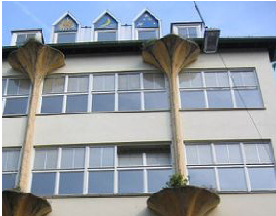
Figure 38. Innovative ways to provide green infrastructure within buildings will be investigated, the example above slows the water on its path to the stormwater system by using planting.
