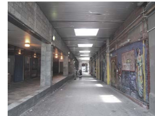
Figure 13. Existing Opera House Lane.
