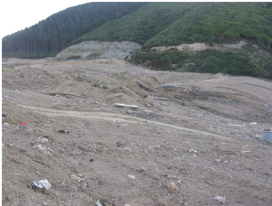
Figure 12: Front face after stripping vegetation. Note leachate discharges (dark strips) 2010
