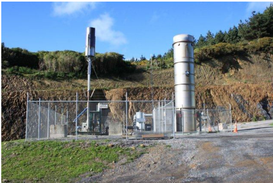
Figure 8: New Gas Flares (Primary & Backup) serving entire landfill (2012)
