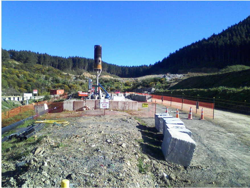
Figure 7: Small gas flare serving old weigh station and kiosk (2006)
