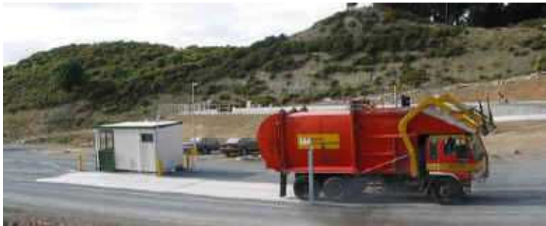
Figure 16: Original kiosk and weigh station built on refuse in 2002
