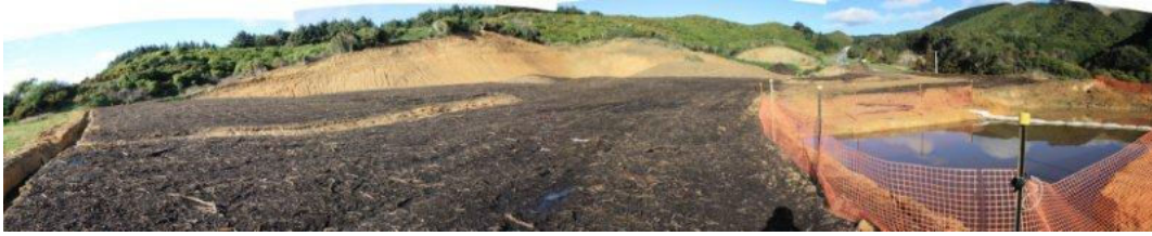
Figure 18: Lower Borrow Area (August 2012)
