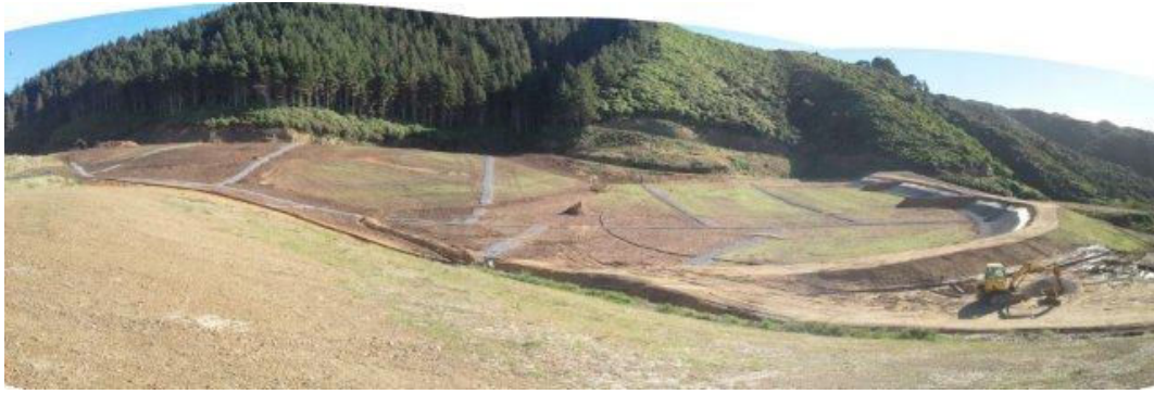
Figure 15: Finished Stage 2, Phase 1.1. New cell almost ready for filling (August 2012)
