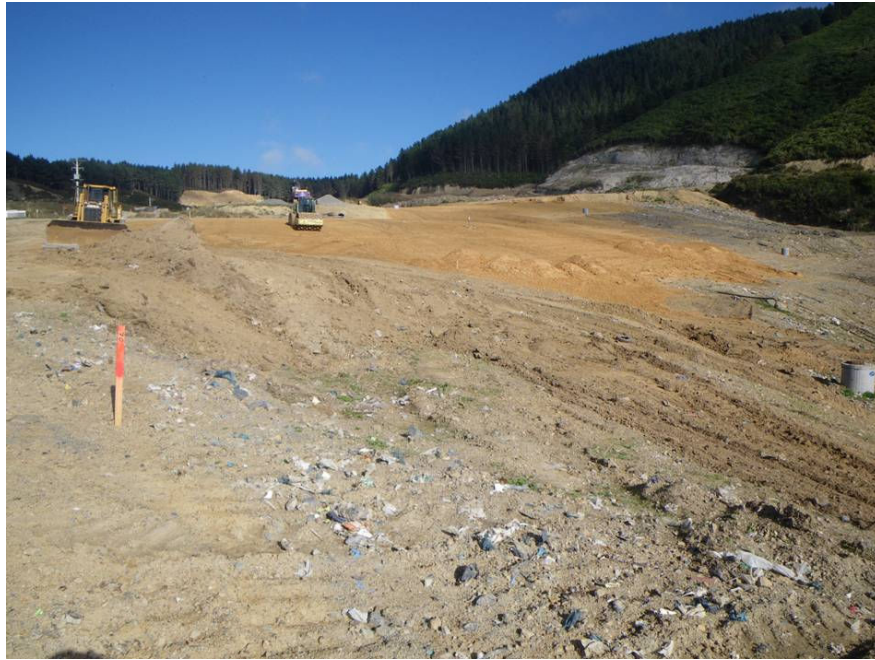
Figure 13: New impervious capping layer to front face 2010
