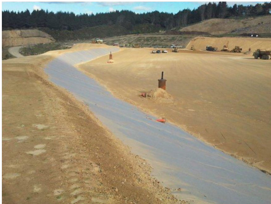
Figure 14: Stage 2; Phase 1.1 - bund, impervious liner and new gas wells 2012
