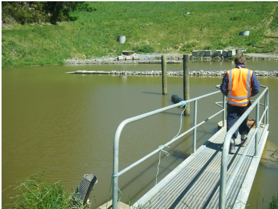
Figure 10: Improved Sediment Pond (2011)
