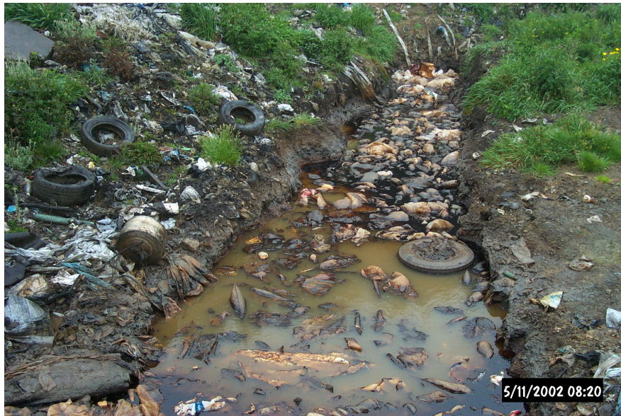
Figure 11: Poor Storm water control creating leachate
