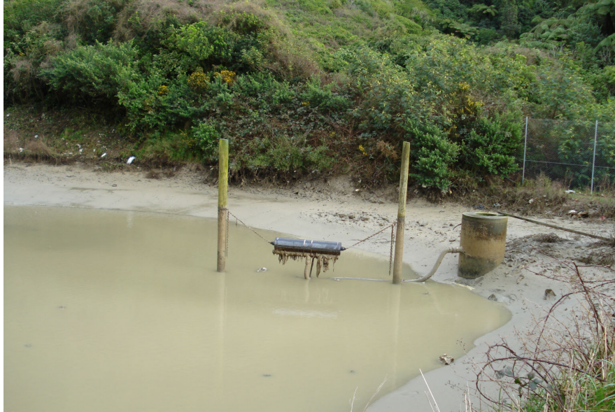
Figure 9: Sediment Pond before improvements (2010)
