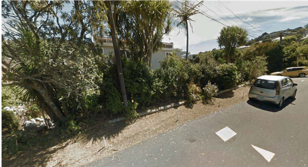
View of road land proposed to be stopped from Woburn Road
