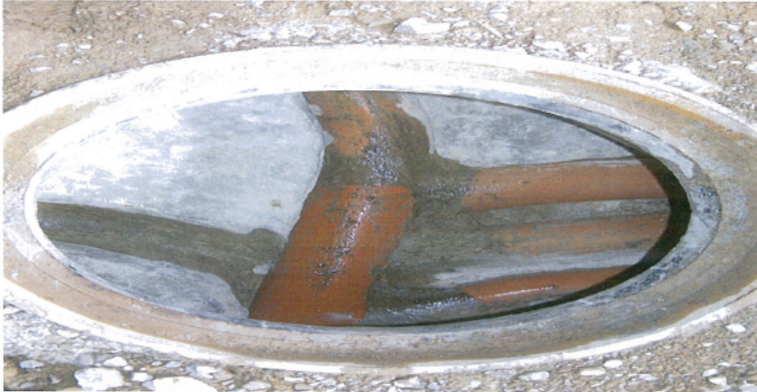
View 2 of manhole with subsoil drain connections
