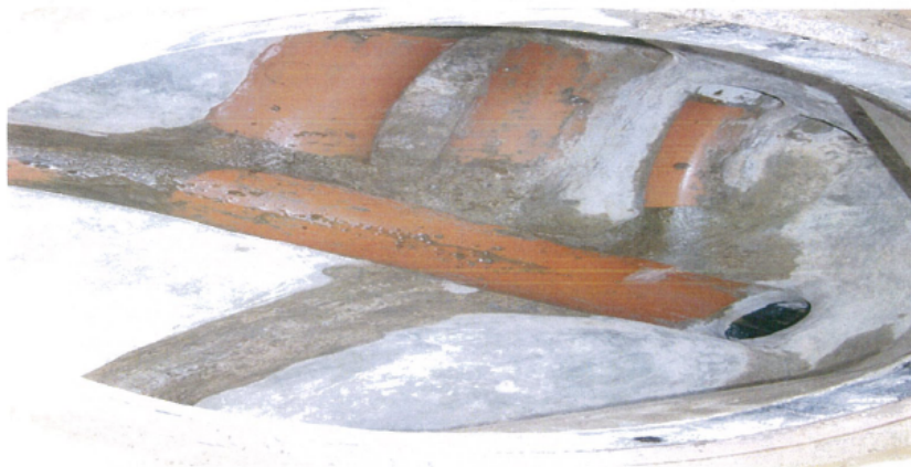
View 2 of manhole with subsoil drain connections
