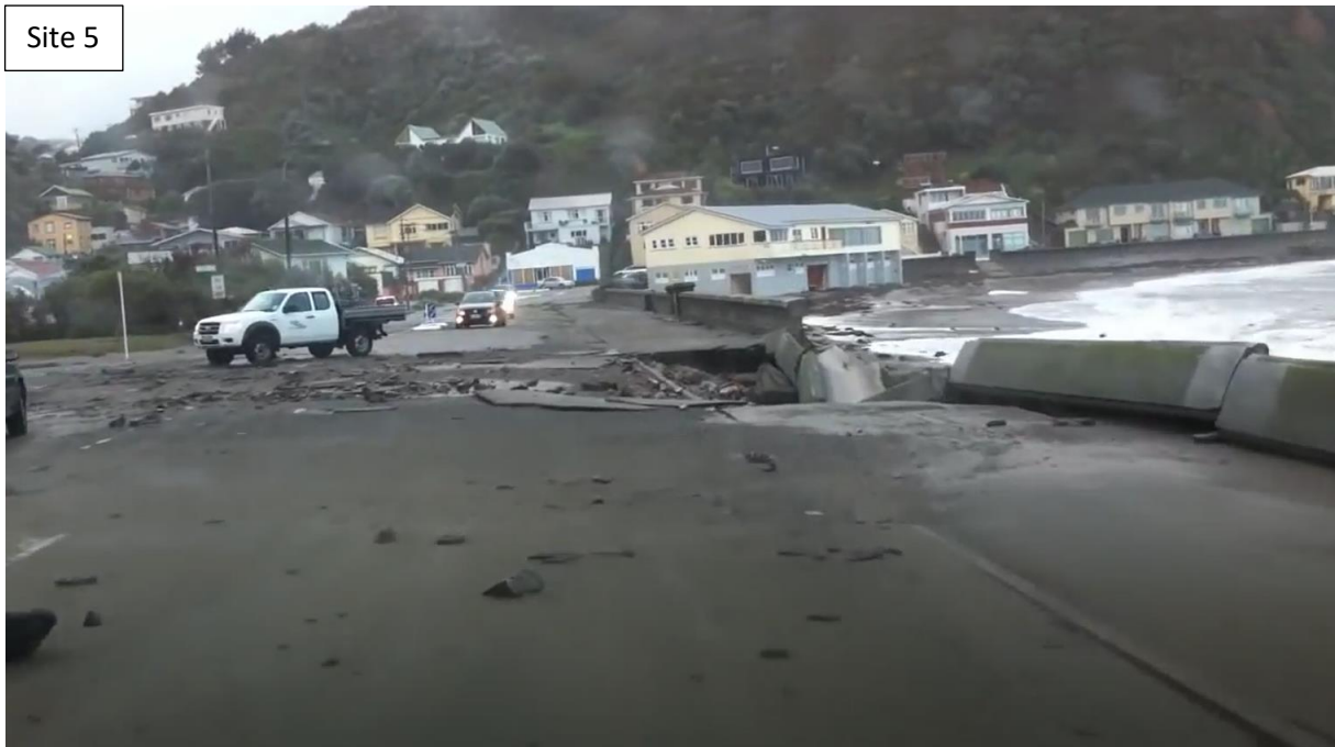
Figure 6-13: Coastal inundation evidence and debris line at site 5 in Figure 6-12. [Source: NIWA New Zealand ].
