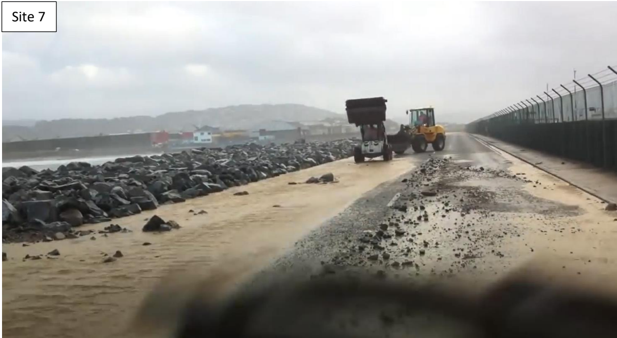
Figure 6-17: Coastal inundation evidence and debris line at site 7 in Figure 6-14. [Source: Wellington City Council ].
