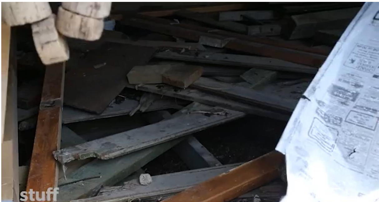
Figure 6-37: Damage presented in Figure 6-36 from the inside of the shed. https://www.stuff.co.nz/environment/110423337/wellington-seaside-village-hatches-climate-change-plan-after-cyclone-gita-mayhem .
