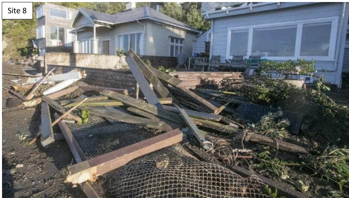
Figure 6-20: Coastal inundation evidence and debris line at site 8 in Figure 6-19. [Sources: https://www.stuff.co.nz/dominion-post/news/121145008/two-days-warning-for-massive-wellington-waves-but-nobody-raised-alarm ].
