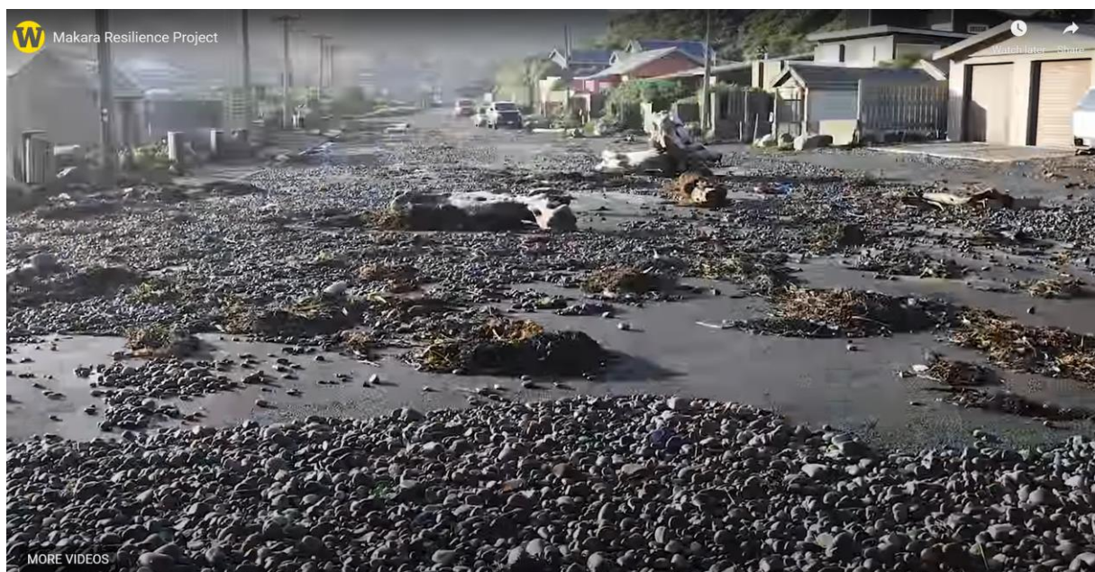
Figure 6-35: Debris in Mākara road. [Sources: https://Mākara-wcc.opendata.arcgis.com/ ].
