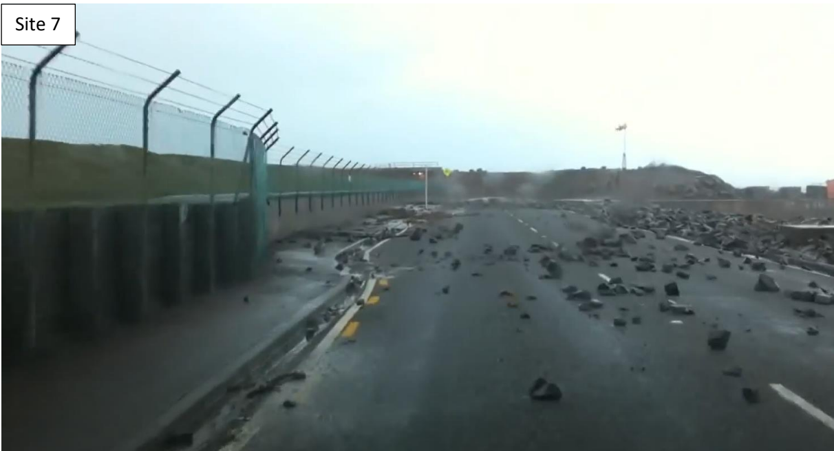
Figure 6-16: Coastal inundation evidence and debris line at site 7 in Figure 6-14. [Source: Wellington City Council ].
