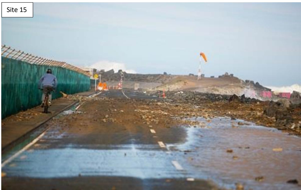
Figure 6-30: Coastal inundation evidence and debris line at site 15 in Figure 6-28. [Source: https://wellington.govt.nz/news-and-events/news-and-information/our-wellington/2020/04/big-waves-hit-wellington-coast ].
