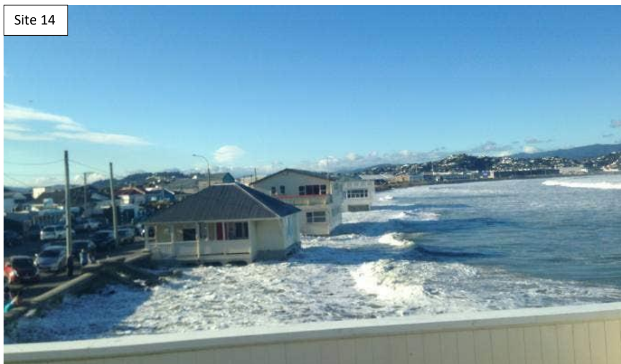
Figure 6-29: Coastal wave runup evidence at site 14 in Figure 6-28. [Source: https://www.stuff.co.nz/dominion-post/news/74187528/rising-seas-a-slowly-unfolding-red-zone ].
