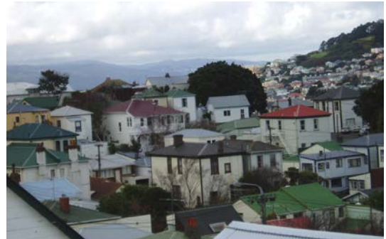
Intricate roofscape demonstrating consistency of roof type and pitch
