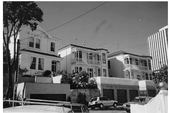
Western side of Portland Crescent – larger set backs and garages built to the street boundary
