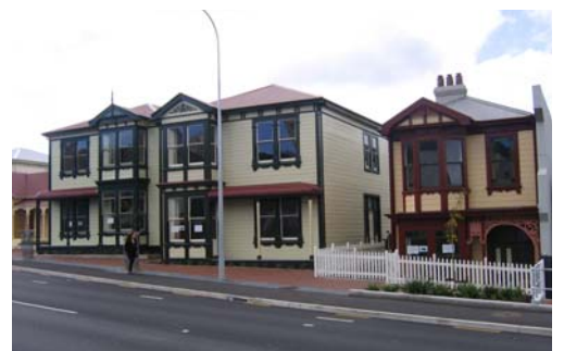
No parking between buildings and the street frontage
