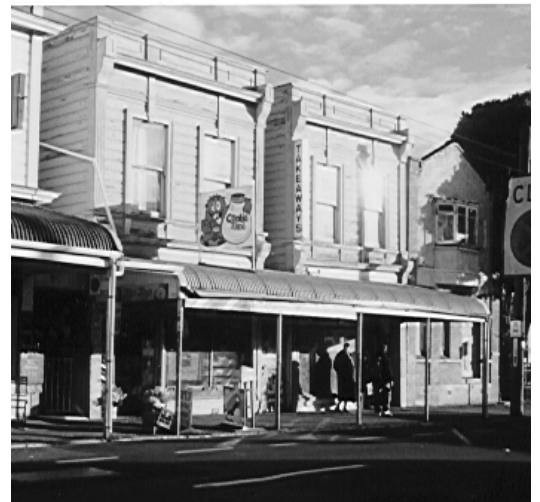
Typical upper Willis Street retail
