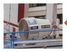
The 'Dust Fighter' provides highly effective dust control and was used successfully recently further up the Terrace on the Mayfair House Annex demolition.
