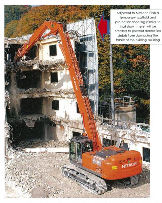
The High-Reach excavators have transformed the way in which demolition of structures is undertaken today. They provide a safe, relatively quiet (reduces overall site noise levels by up to 10dB) and effective means of minimising the effects of demolition especially to neighbouring properties.
