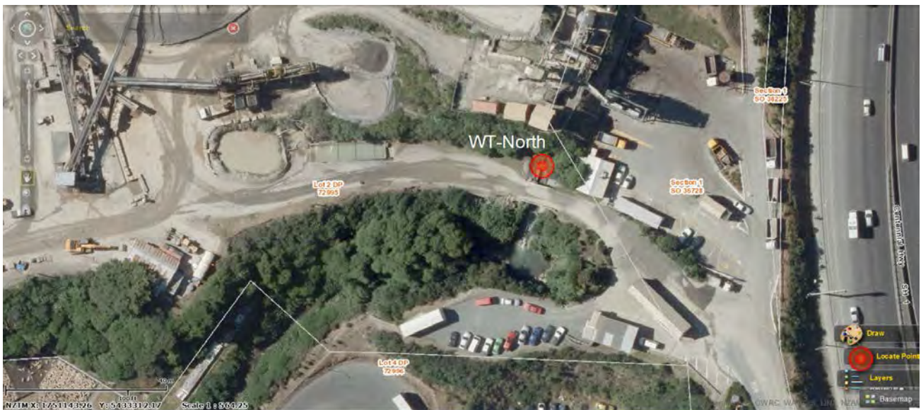
Figure 2-1: Location of the existing water take for the northern quarry face (WT-North)
