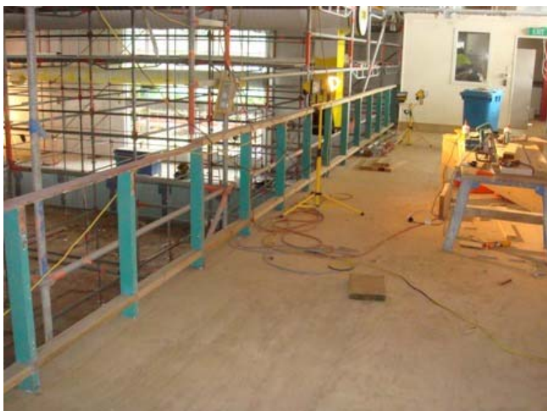
View from the mezzanine in the pool, March 2012.
