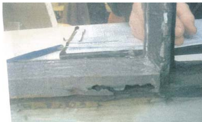
The building (left) and an example of the window frame corrosion (right).
