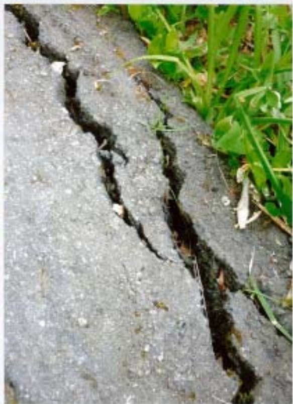
Sections of the common access path to the Salisbury Court Garden Heritage Area, showing subsidence and path damage. Glazed drain tiles will be replaced and realigned after the retaining walls are built and as the new asphalt path is laid.
