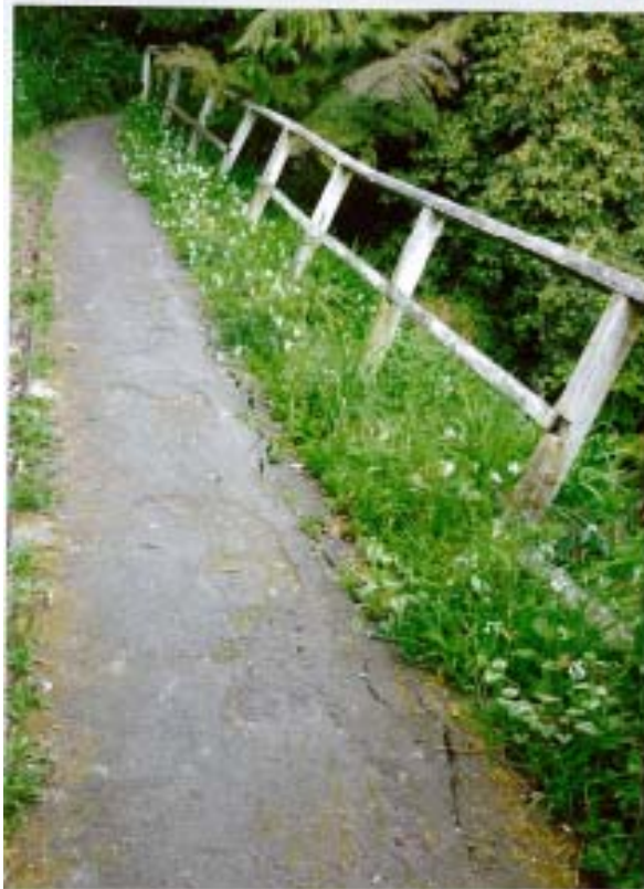
Sections of the common access path to the Salisbury Court Garden Heritage Area, showing subsidence and path damage. Glazed drain tiles will be replaced and realigned after the retaining walls are built and as the new asphalt path is laid.
