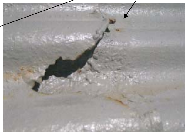
Gutter and roof corrosion
