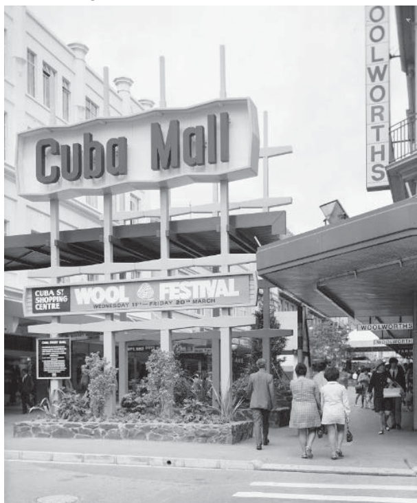
Cuba Mall entrance, Wellington. Winder, Duncan, 1919-1970 :Architectural photographs. Ref: DW-4160-F. Alexander Turnbull Library, Wellington, New Zealand. http://natlib.govt.nz/records/23118555
