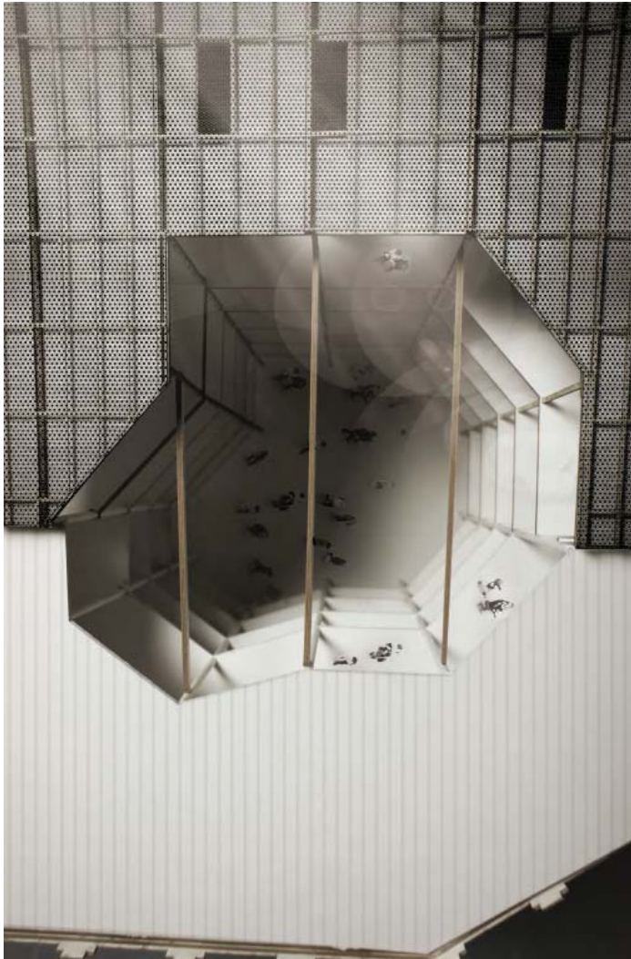
View of void. The junction between the old and new building parts and the expressed contrast showing co-dependence of both.
