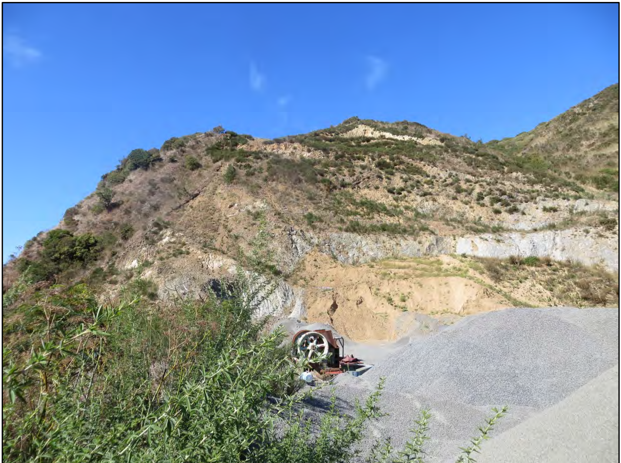
Figure 1-6: Photograph of the Kiwi Point Quarry Southern Ridge Looking South
