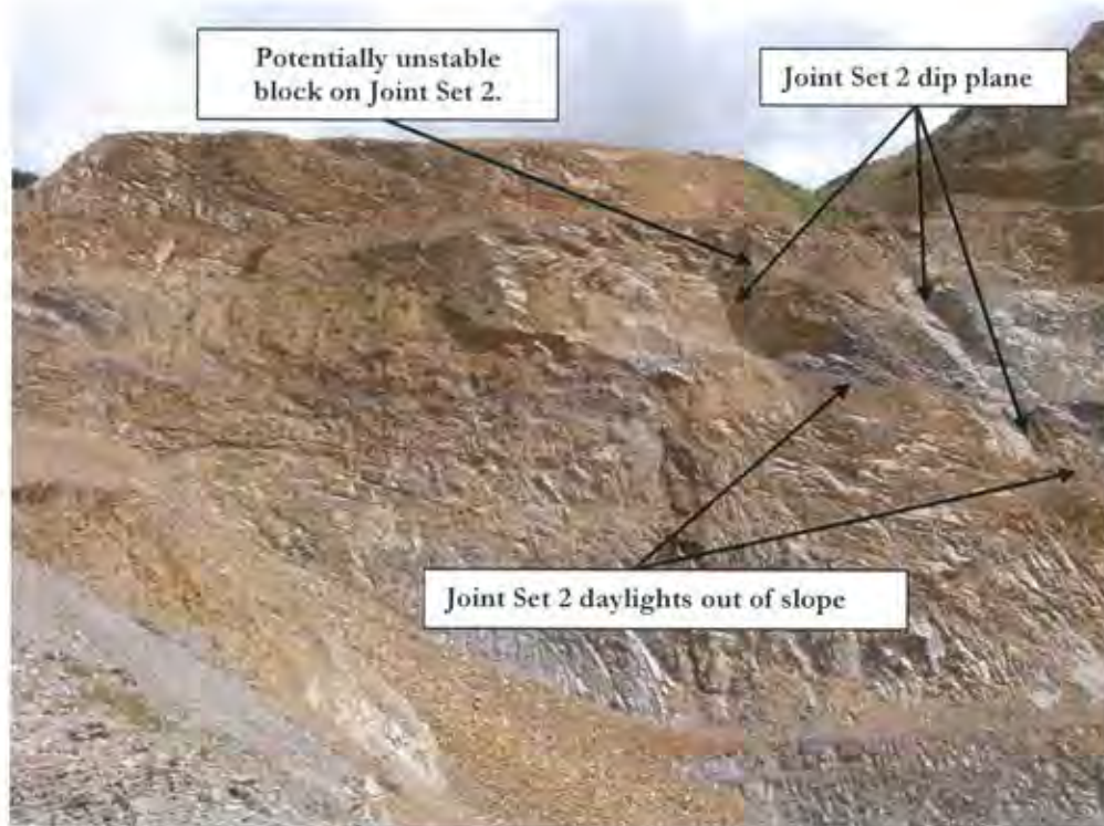
Plate 6 View to the west of the western batter showing Joint Set 2 dipping out of the face and remnant undermined kinematically unstable blocks perched on the batter slope.
