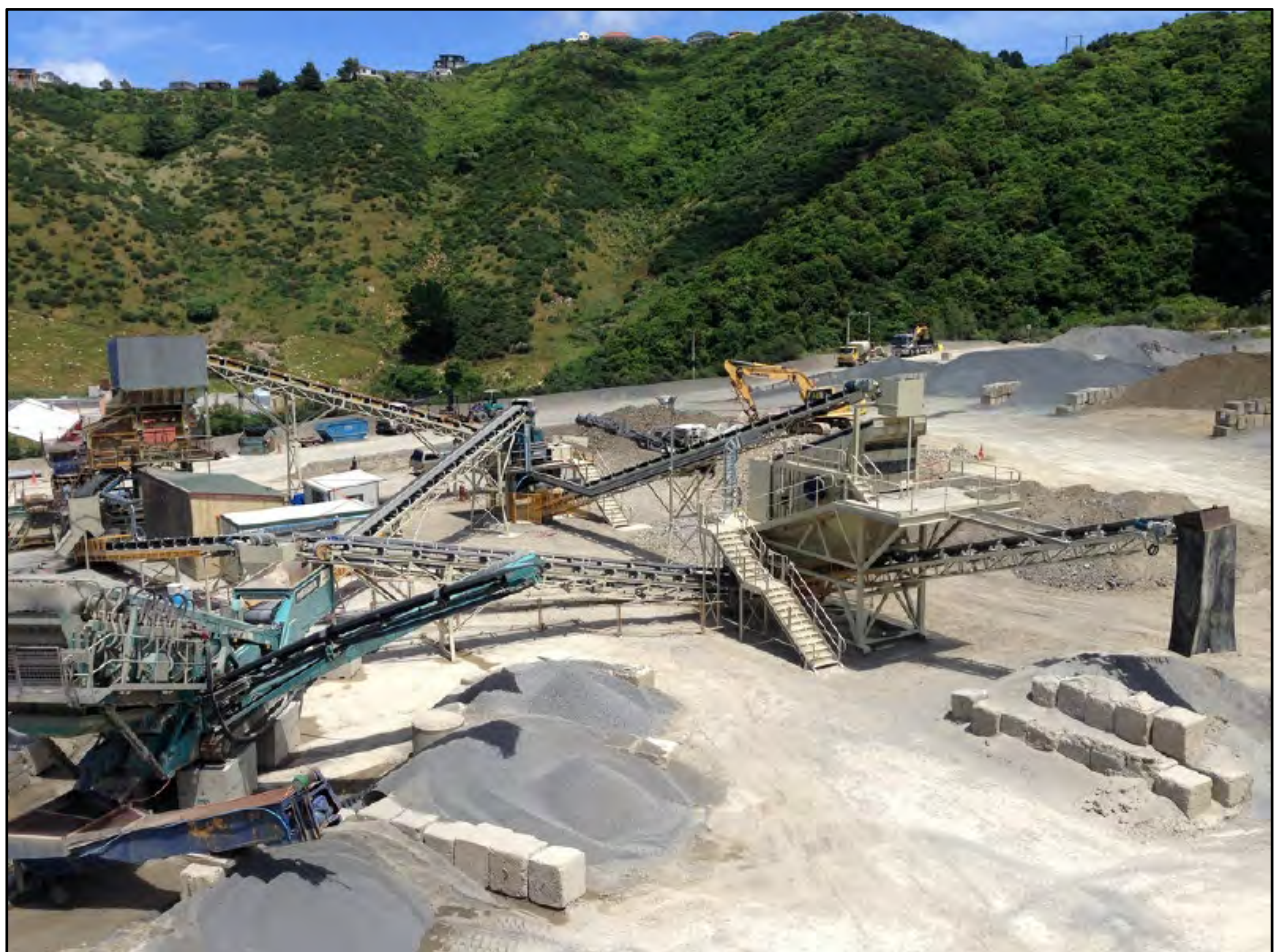
Figure 1-5: Photograph of the Kiwi Point Quarry Processing Plant at its Existing Location
