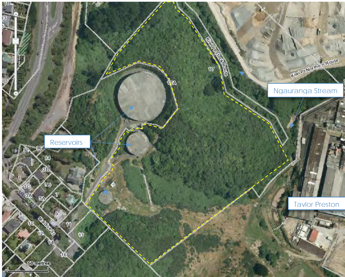
Figure 2: General location of Area 1A showing key features (Base image source: WCC webmap).
