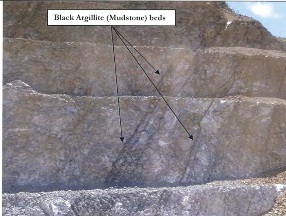
Plate 2 Northern Batter exposing slightly weathered to fresh sandstone dominant greywacke with bedding dipping to the left as defined by black argillite beds.
