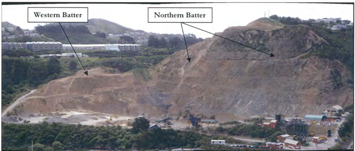
Plate 1 General view of Kiwi Point Quarry looking to the Northwest with the main northern batter at the right and western batter at the left.
