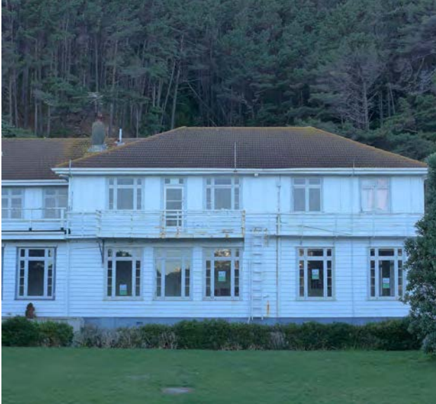
BUILDING 07 Fig: DG 2.3.2
