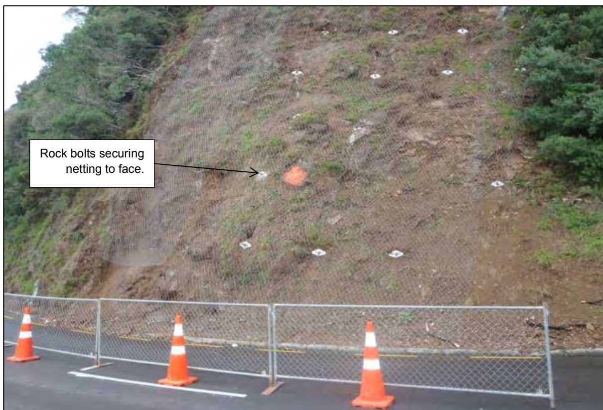
Figure 9 Rock netting designed by AECOM and installed on Birdwood Street, Wellington, 2013.
