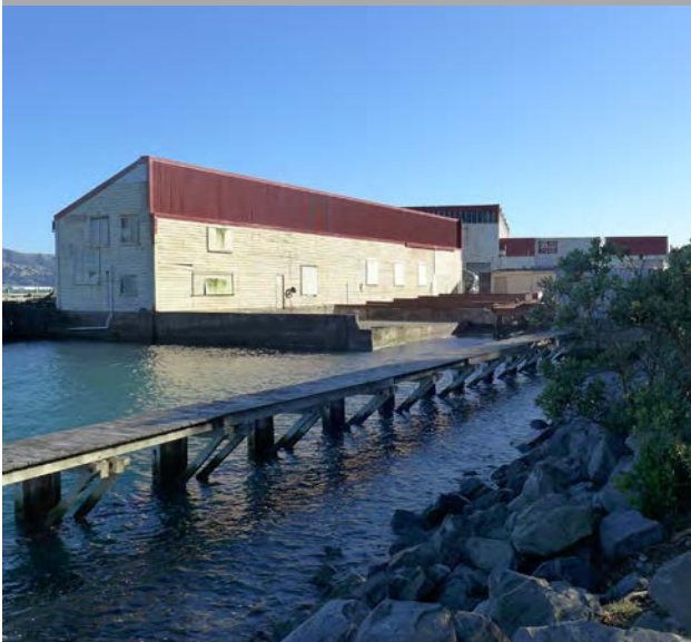
BUILDING 12 Fig: DG 2.3.3
