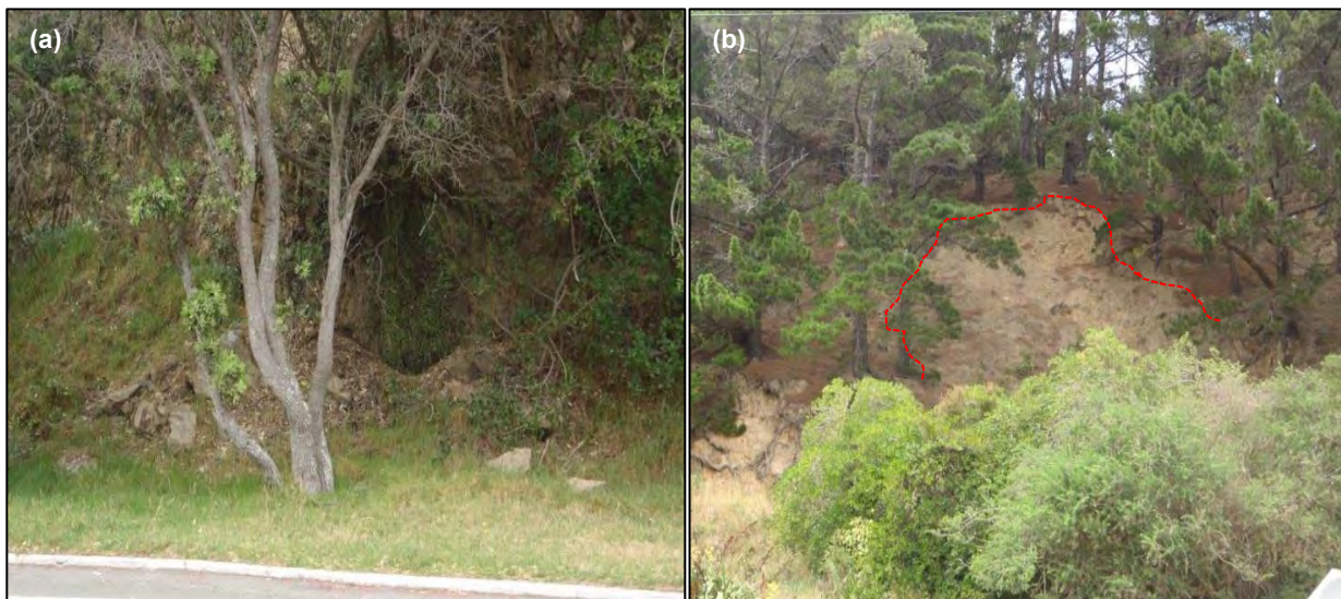
Figure 6 (a) Rock fall debris at toe of Slope 5; (b) Extent of shallow surface failure above greywacke outcrop at Slope 8
