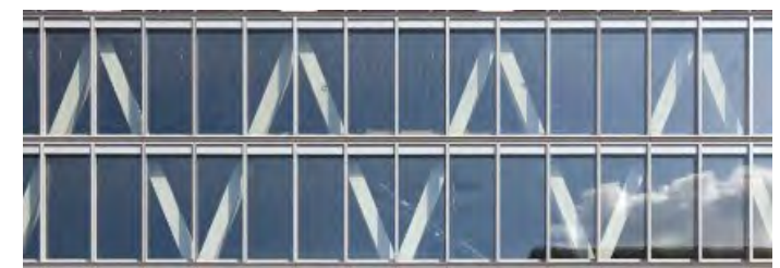
Exposed Gantry Structure - ABR building, Rotkreuz, Burckhardt & Partner AG
