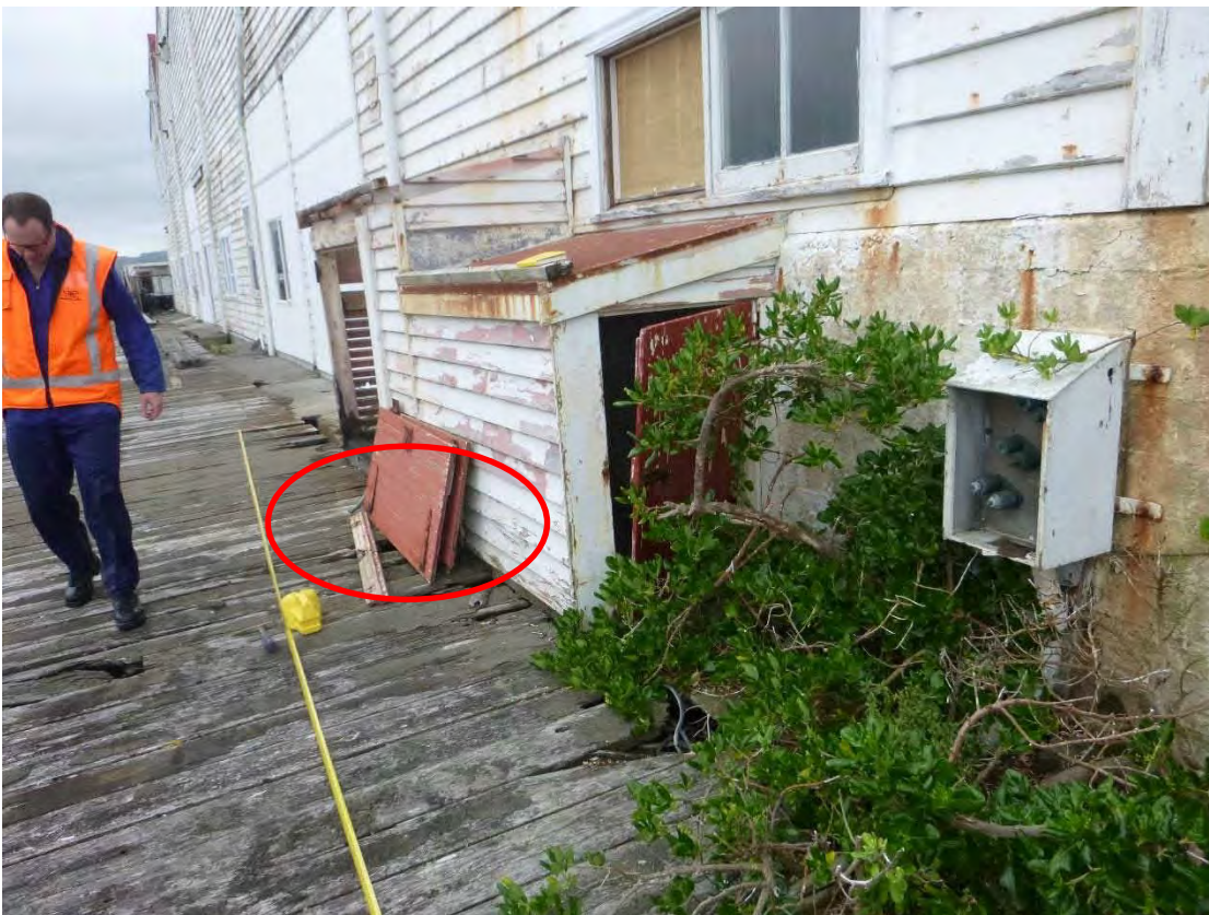
Photo 6. Access to critical foundation No. 2.
