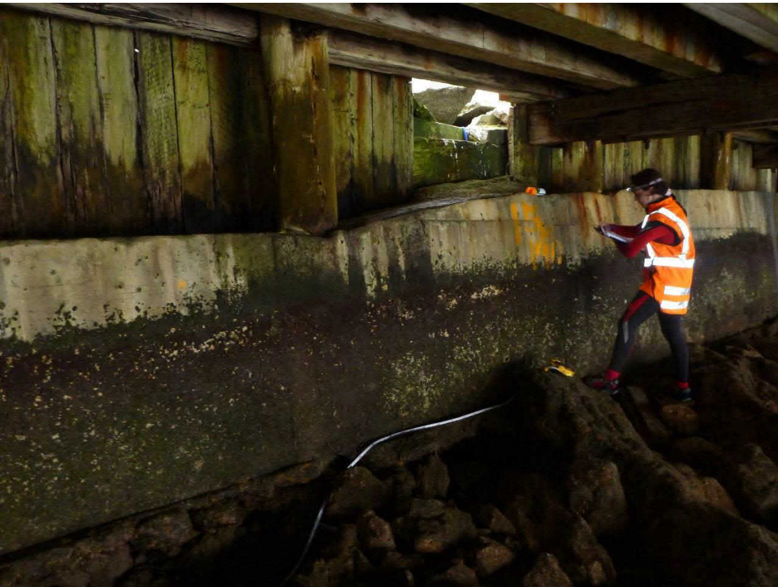
Photo 2. Access to critical foundation No. 1 from water
