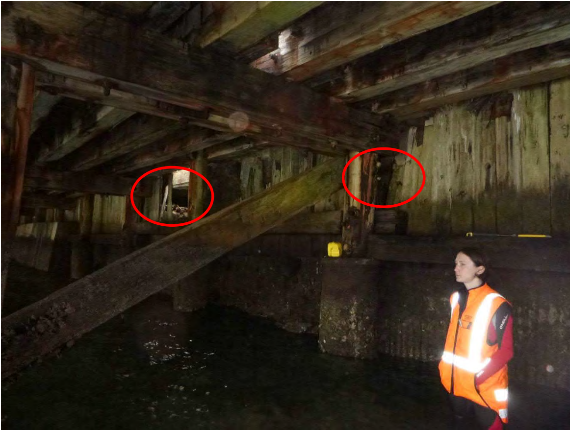
Photo 7. General overview for access to critical foundations from water.
