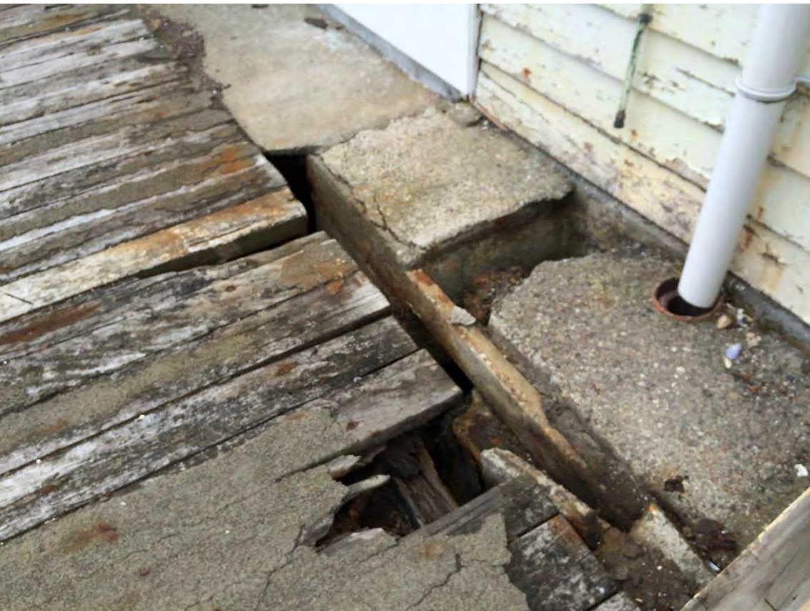
Photo 4. Access to critical foundation No. 1.
